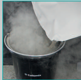
While filling the bucket, a large amount of dust is produced.
